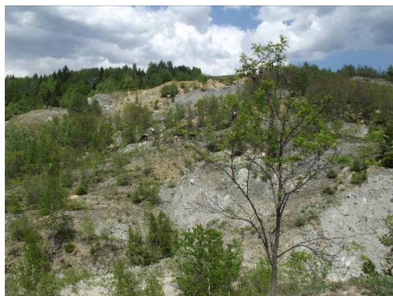
Fig. 2. Plastic flows on the quarry's slopes
