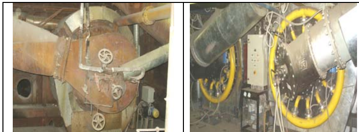
Fig. 7 – Burners with reduced NO x for unit no. 3.
